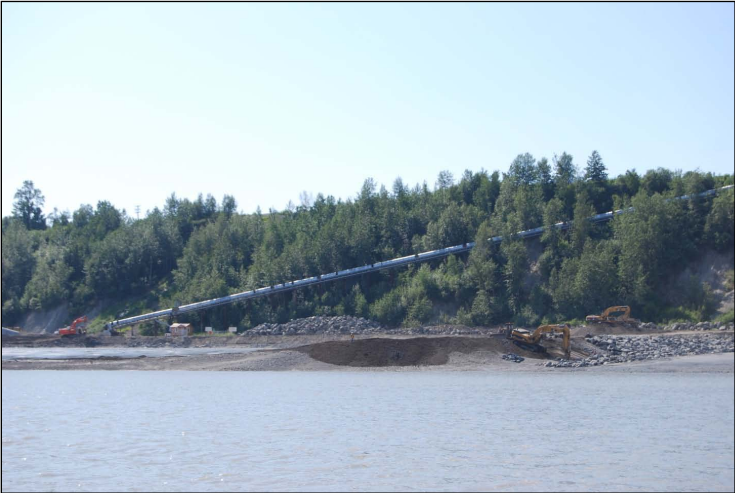
Figure 16. On-land construction activities at Port MacKenzie during July 2010.
