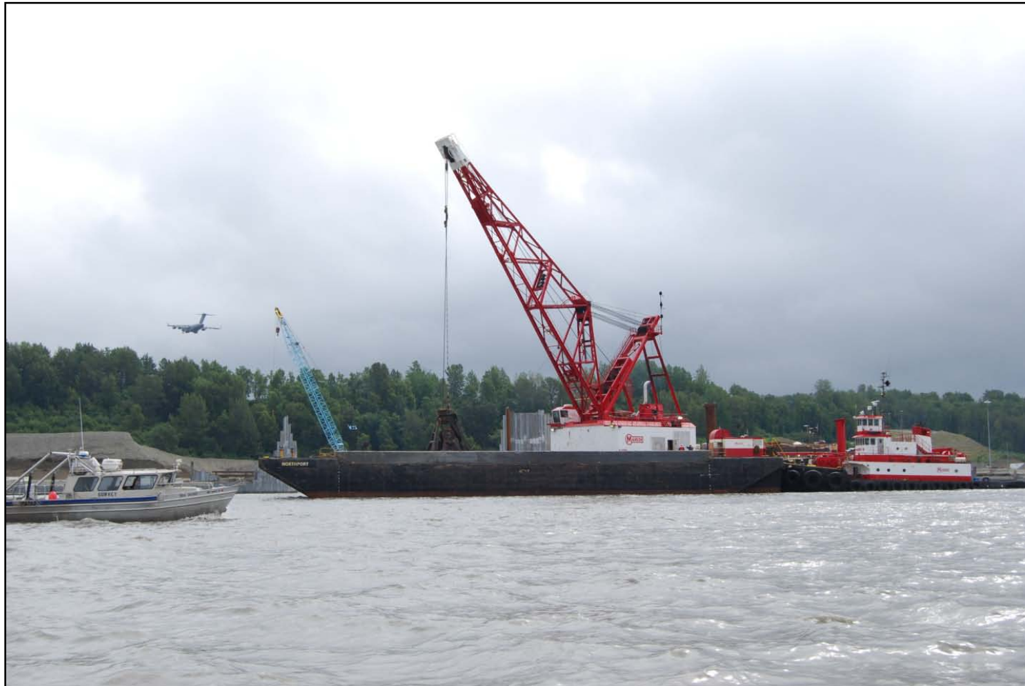
Figure 15. Example of multiple noise sources operating concurrently near the Port of Anchorage, which contribute to ambient noise conditions of Knik Arm.
